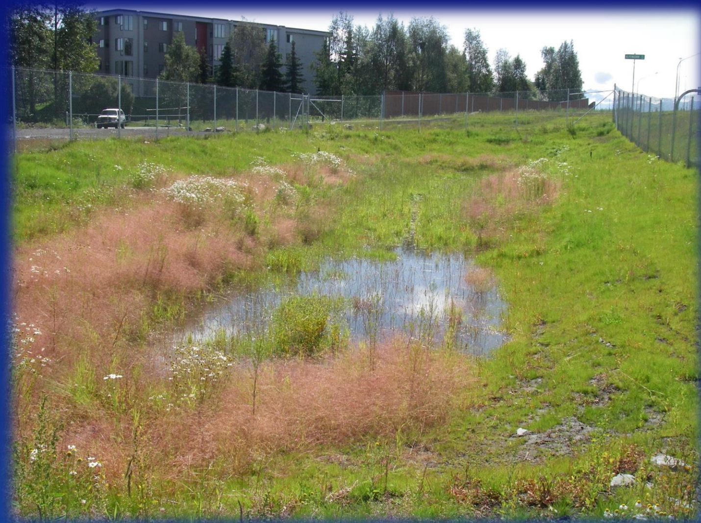
NSH Infiltration Basin
